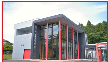
New Kakuda factory in Miyagi, Japan
